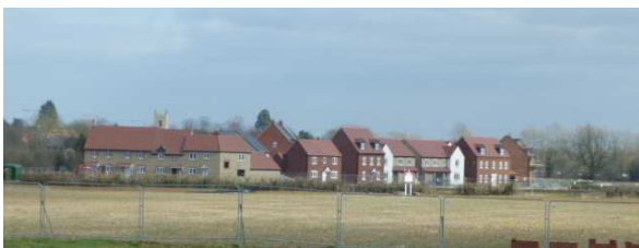
Kingsmere, Bicester, where we were involved in the scheme design from the master plan through Design Code to detailed design with lead developer Countryside properties
