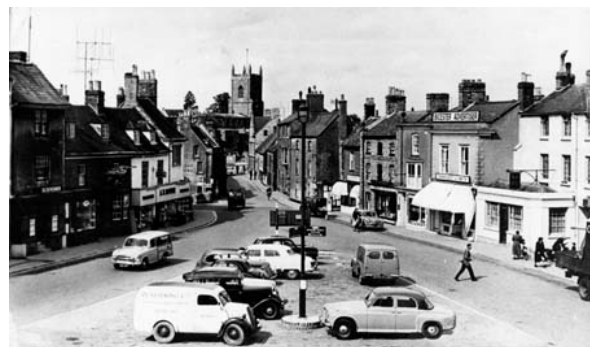
Market Square before the construction of Manorsfield Road. Notice how the space funnels views towards the Parish Church (below)
