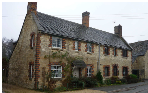
Springdale & Bishop's Cottage, non-designated heritage assets in Kirtlington; former Estate cottages where the window and door openings are framed in local red brick, with the burnt headers creating an attractive chequer board effect, that is highly locally distinctive
