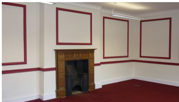
Interior of Old Bodicote House, refurbished, following guidance from the Team
